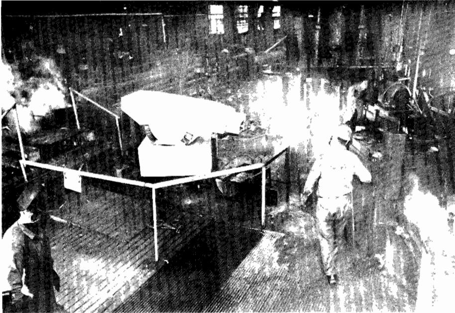
**Figure 2-7.** A Unimate robot similar to the first servo-controlled industrial robot, working in a hazardous industrial foundry application. This robot is unloading hot ingots from a furnace. (Courtesy of Joseph F. Engelberger.)
