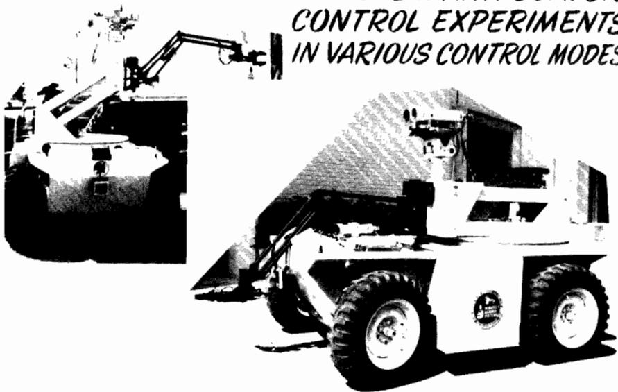
**Figure 2-2.** Remote manipulators in experiments in various control modes. Top left: a slave manipulator equipped with stereo cameras. Bottom left: A mobile manipulator equipped with grippers and camera systems. Top right: The control boards showing the monitors for camera viewing, and the joysticks and switches for manipulator control. Bottom left: A side view of the mobile manipulator. (Courtesy of JPL/NASA.)
