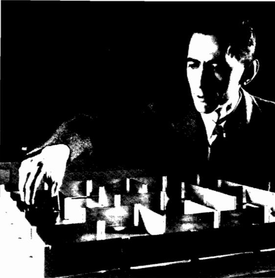
**Figure 2-6.** Claude Shannon is shown here with his robot mouse, which could navigate a maze of 25 squares in 15 seconds. The robot “learned” its way through the maze after a 2-minute trial-and-error run. (Courtesy of the Massachusetts Institute of Technology Museum, Cambridge, Massachusetts.)
